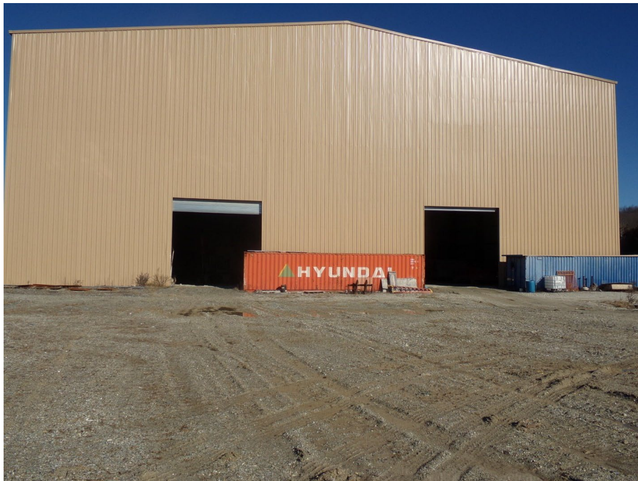
Exterior of Building 2 (Western Side of the Building)
