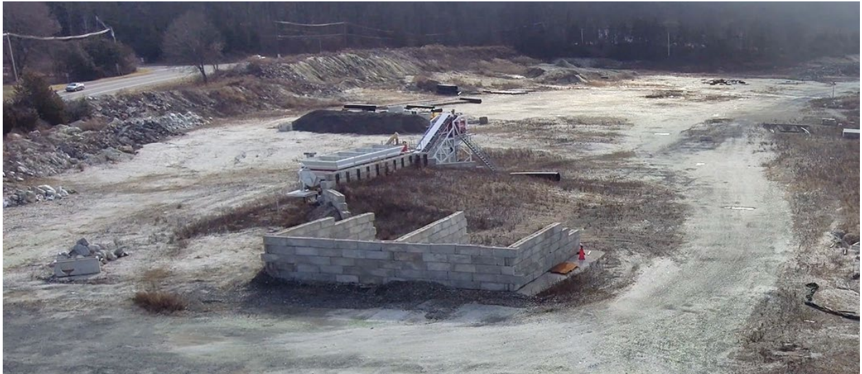
Assembled Concrete Block Structure and Portable Concrete Plant
