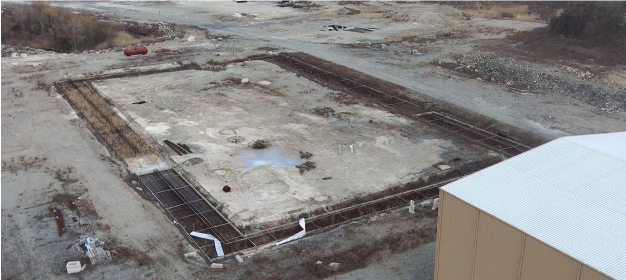
Views of the partially constructed foundation of Building 1.
