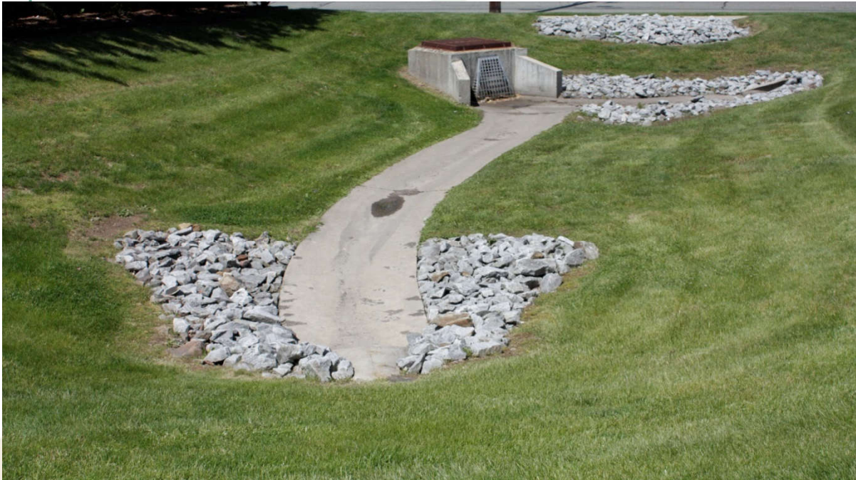
A well-maintained detention basin
