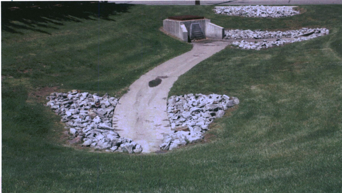
A well-maintained detention basin
