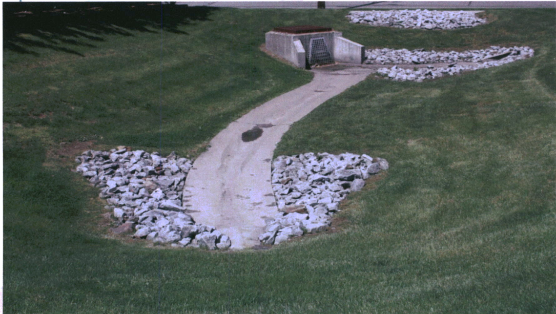
A well-maintained detention basin
