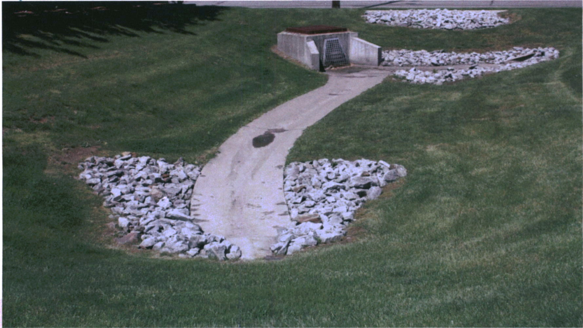
A well-maintained detention basin
