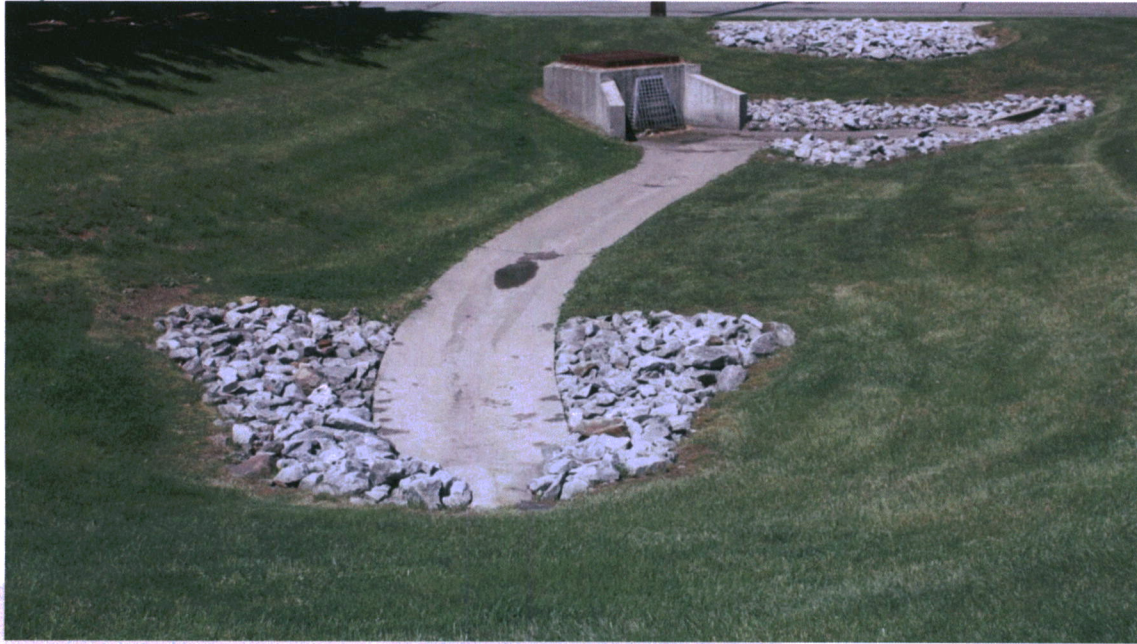
A well-maintained detention basin
