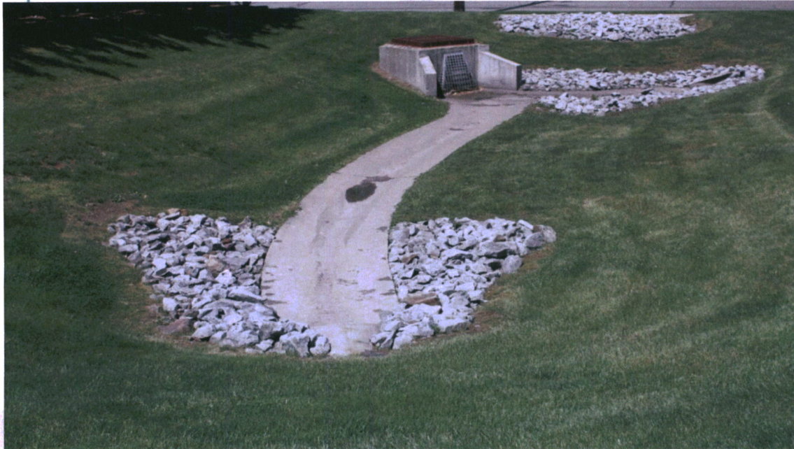
A well-maintained detention basin
