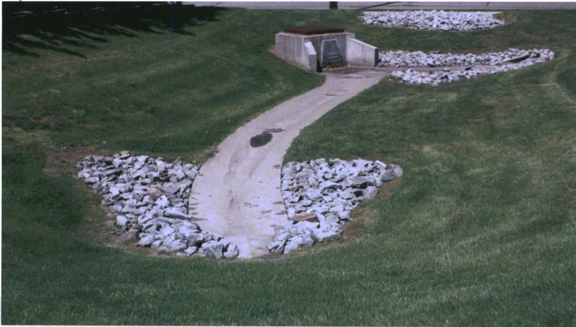
A well-maintained detention basin
