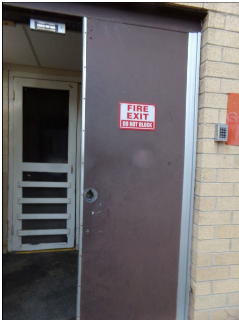
Broken handle on fire exit.
